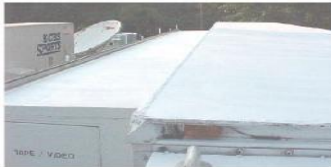
Coated Exterior Roof
